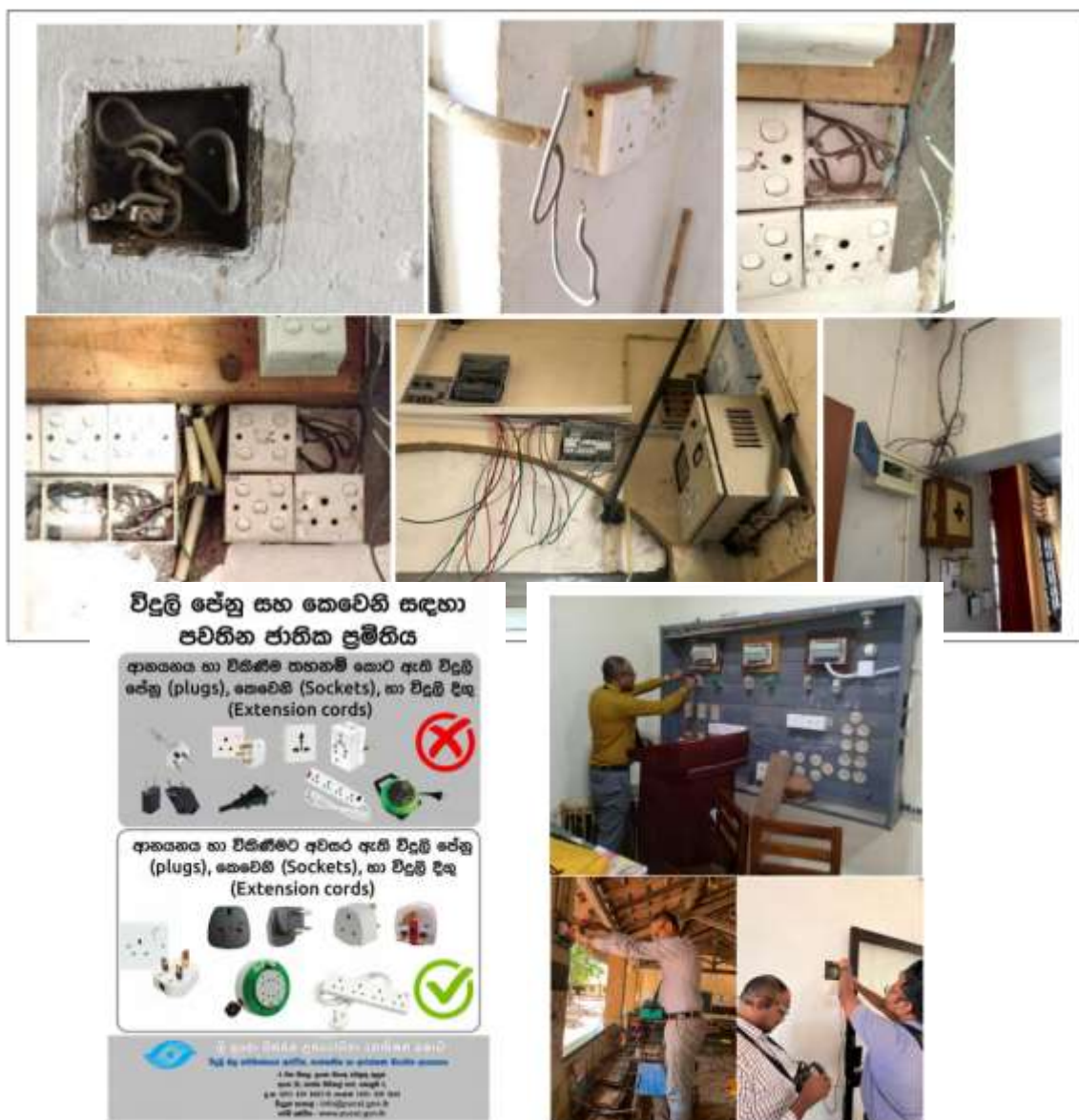
Figure 8 Inspection of Unsafe wiring practices was common, with open-ended wires, disconnected earth conductors, and unsecured cable runs frequently observed
