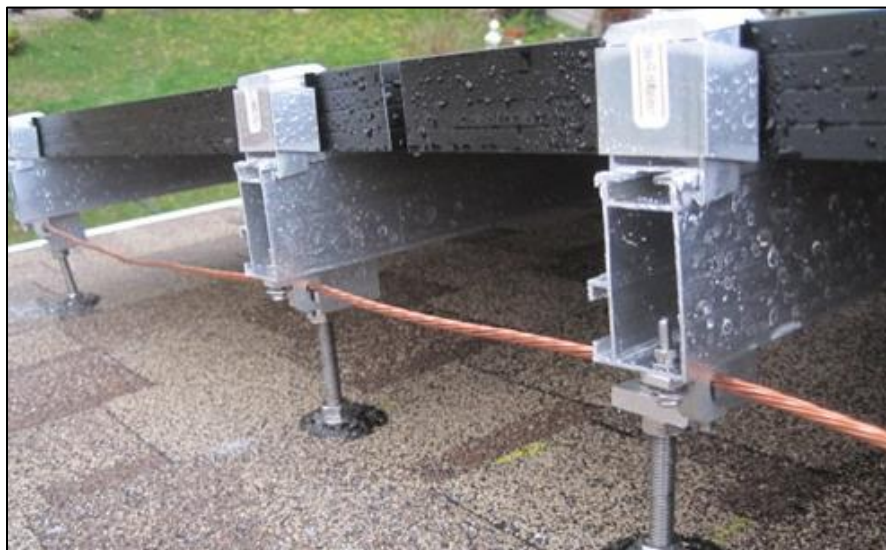
Figure 3-2: Earthing of PV Modules
