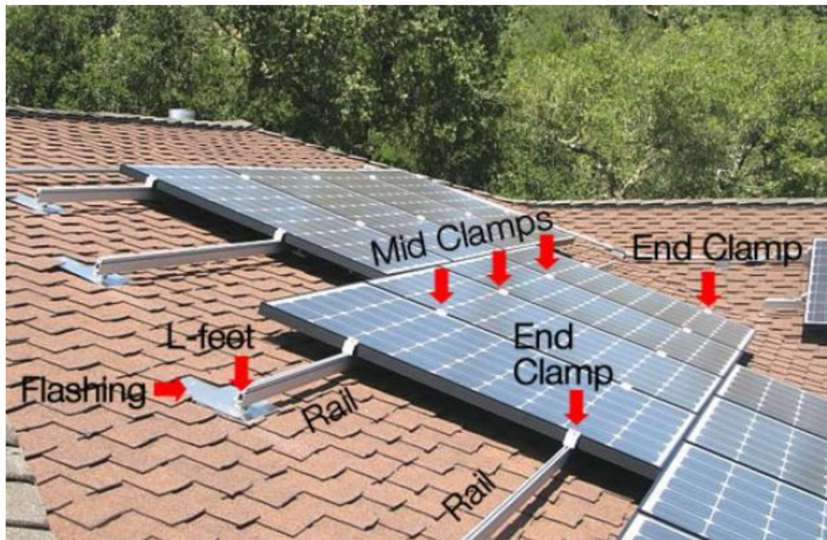
Figure 4-1: Mounting arrangement of PV panels
